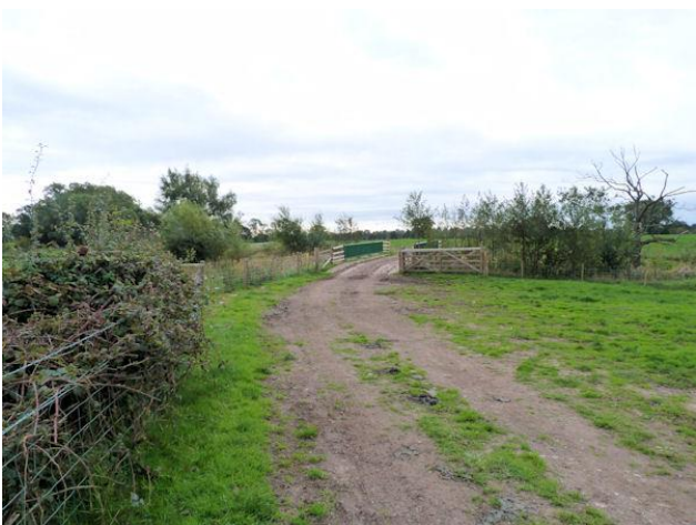
Bridge over River Dean at boundary of Woodford
